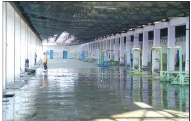
Improved condition of Veraval fishing harbour
