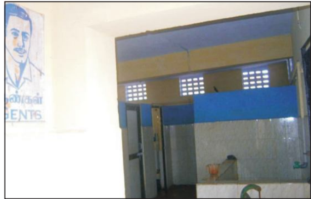
Reopened Toilet at Kasimedu harbour
