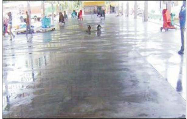
Improved condition of Thopumpady fisheries harbour
